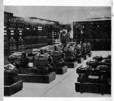
Motor generators (above) develop the power used. Stored in batteries to assure a smooth, uniform flow, the reserve could run Radio City for 72 hours!
